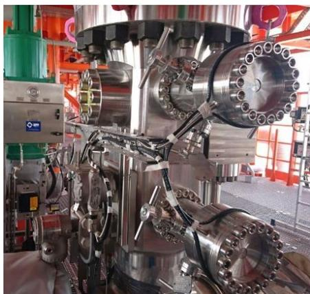
Figure 2: VX MPFM installation on unmanned island
